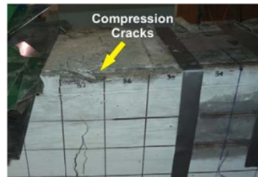
Fig. 10 Typical Failure on Concrete Compression
